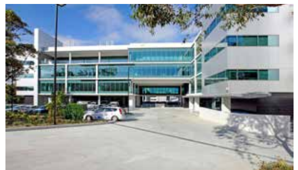
NMI's North Ryde Facility.
